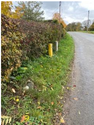
Current utilities in verge
